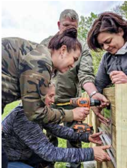
Volunteers work together to construct the gaga ball pit.
