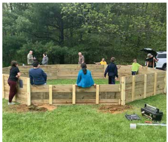
The gaga ball pit frame is almost completed.
